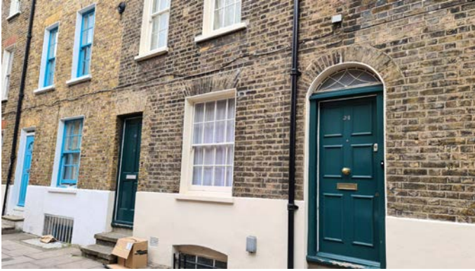
This is what 34 Parfett St looks like now, after refurbishment
