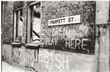
Children in the Parfett Street area play in hazardous traffic conditions.
